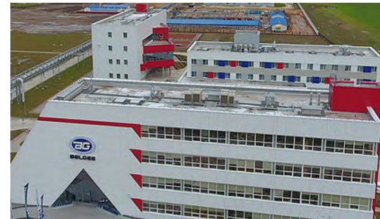
Construction of the automobile plant Belgee" Belarus
